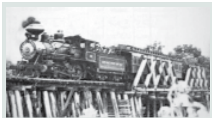
The LOP&G wooden trestle over the Suwannee River. This structure is present on Dr. Butler's layout and still standing today.
